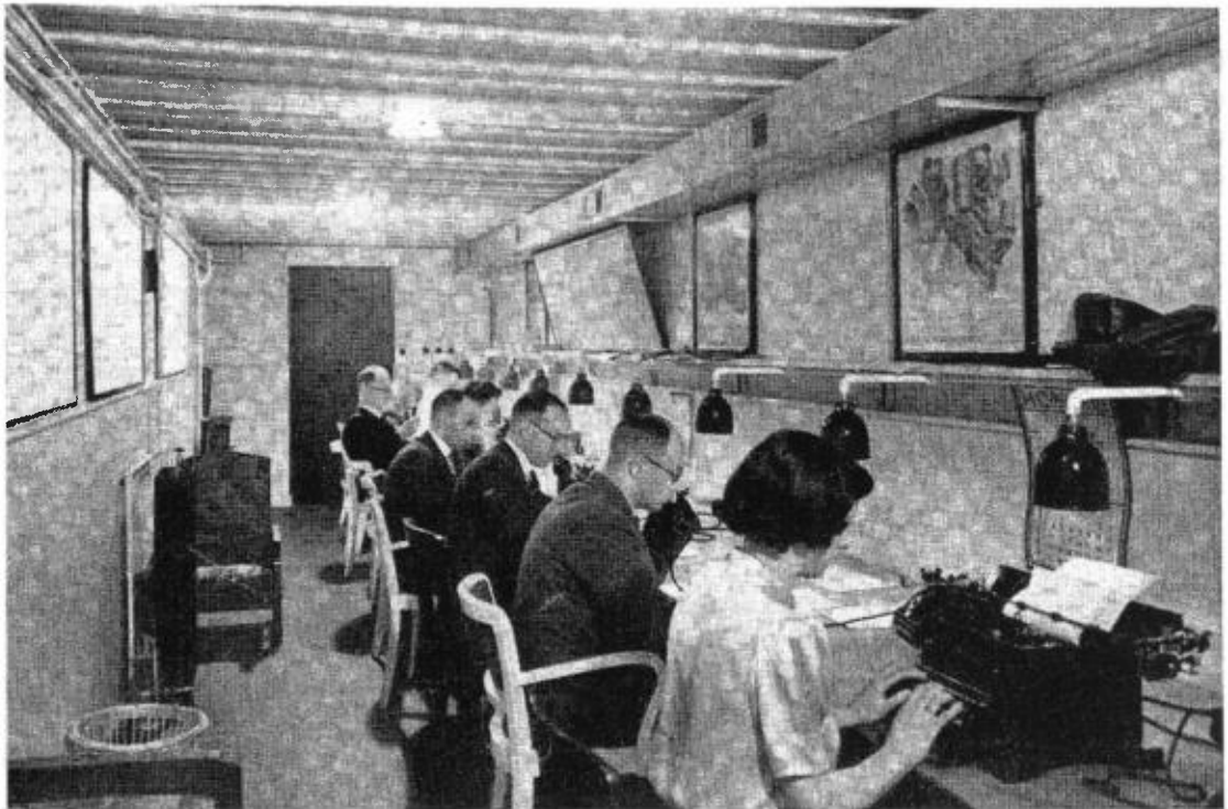
The Control Room
